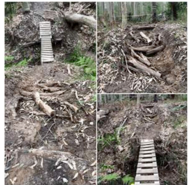
Superbowl's A-Line Bridge pre Trail Crew magic.
