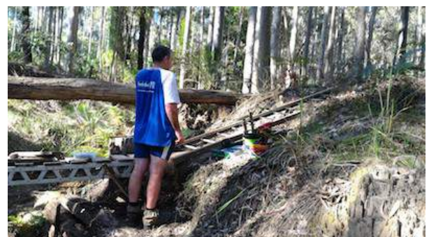
Tony @ Superbowl's A-Line Bridge mmm Where to start?.
